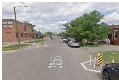
Figure 16: Paint-and-post chicane on 30 th Street in Denver
