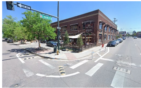
Figure 15: Paint-and-post bulbout on East 13 th Avenue in Denver
